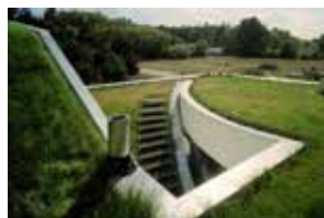
Green Roof and Stair light wells
