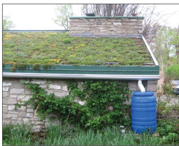
Fig. 1. Sloped green roof at Civic Garden Center of Greater Cincinnati, used for monitoring of runoff water quality on full-scale roof.
