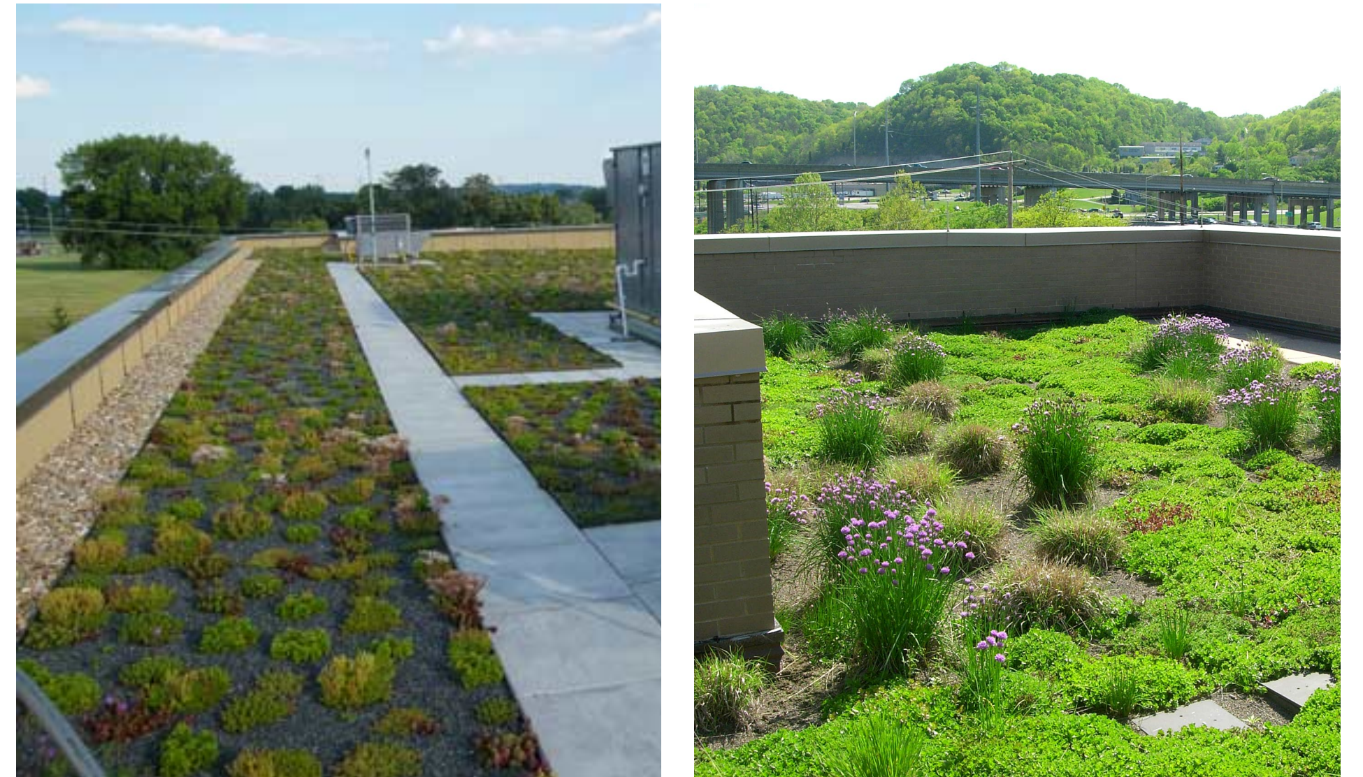
Figure 4: Green Roofs at the Metropolitan Sewer District of Greater Cincinnati (MSD) (left) and Sanitation District #1 of Northern Kentucky (SD1)(right). These sites have monitored stormwater runoff and energy balance of the roofs.
