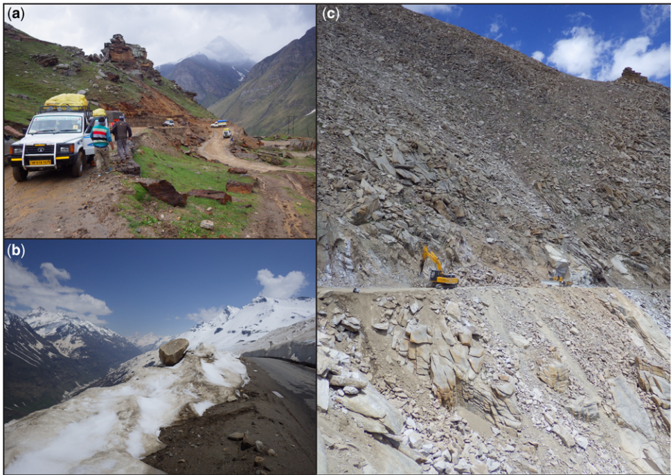
Fig. 8. Human-induced mass movement along highways in the Himalaya illustrated with examples from northern India. (a) Shallow landslide and debris flows during the monsoon season and (b) deep snow drifts and rock-fall debris near the Rhotang Pass in Lahul. (c) Road maintenance underway through thick talus and bedrock slopes at c. 5000 m asl near the Khardungla Pass in Ladakh.
