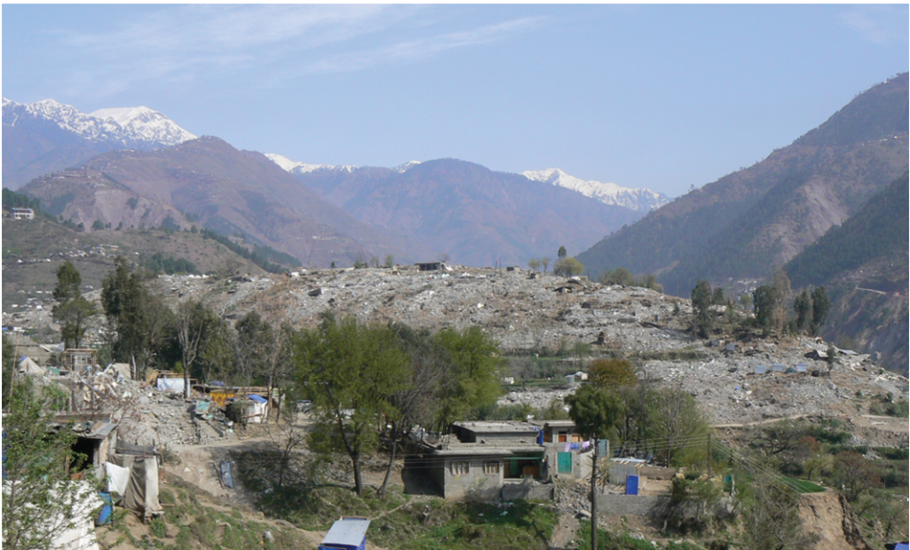
Fig. 3. The remains of the town of Balacot, northern Pakistan that was destroyed by the 2005 Kashmir earthquake; poor building design and location contributed to the catastrophe.
