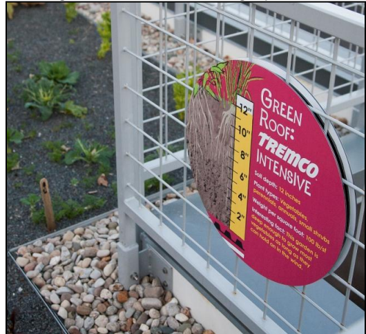
Figure 6: Signage explaining intensive green roof system
