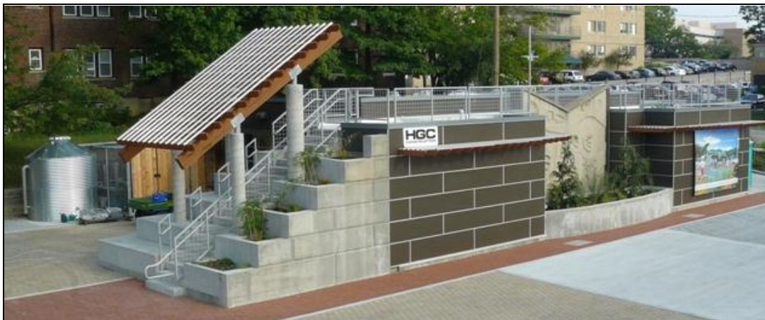
Figure 2: Green Learning Station roof access staircase after construction
